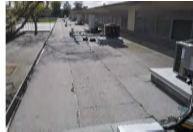
Roof Overview - Building 2 (Buildings 3, 4, and 8 Similar)
