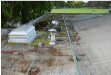
Roof Overview - Building 1
