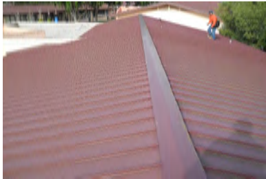
Roof Overview - Building A
