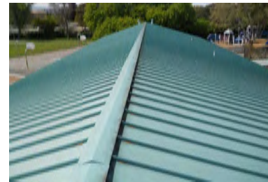
Roof Overview - Building N
