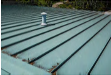
Roof Overview - Building D
