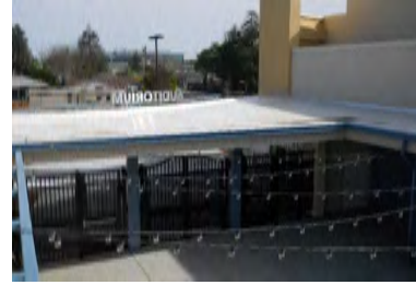
Roof Overview - Building 600
