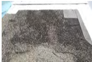
Roof Overview - Building A
