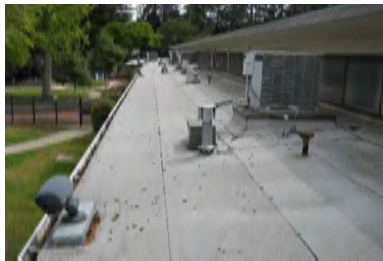
Roof Overview - Building 1&2
