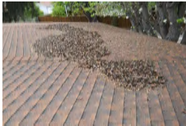
Typical Deficiency - Debris have accumulated on roofs. Recommend clearing debris from all gutters, drains, waterways, and field of roof to promote positive drainage.
