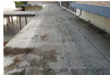
Roof Overview - Building 800
