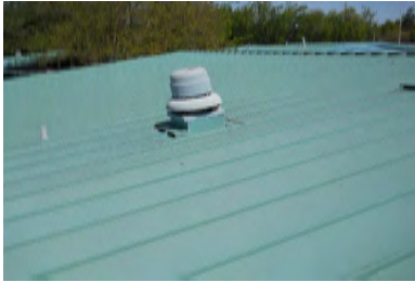
Roof Overview - Building H
