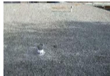
Roof Overview - Building Restrooms
