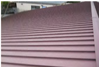
Roof Overview - Building H
