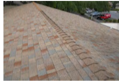
Roof Overview - Building 700
