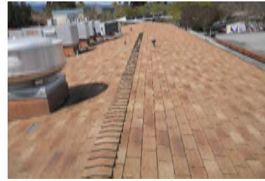
Roof Overview - Building 12
