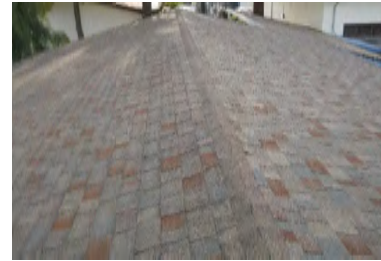
Roof Overview - Building 100
