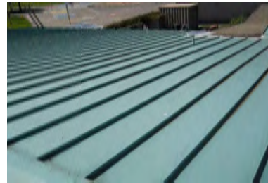
Roof Overview - Building G
