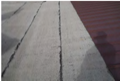
Roof Overview - Building A
