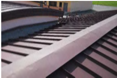
Roof Overview - Building D
