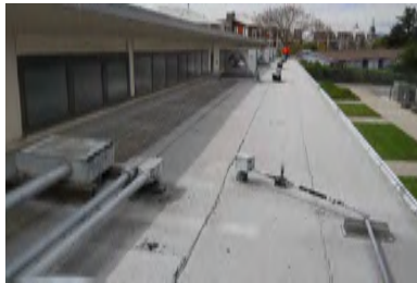
Roof Overview - Building 3
