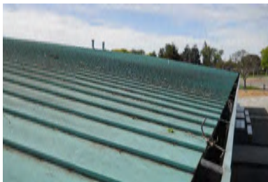
Roof Overview - Building P
