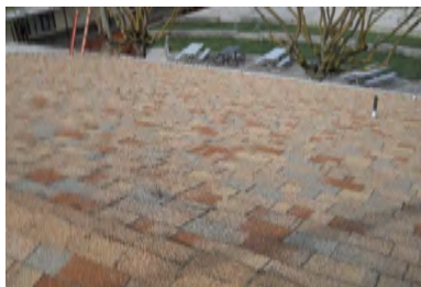
Roof Overview - Building 800
