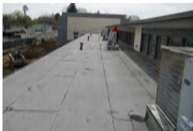
Roof Overview - Building H
