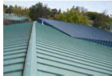
Roof Overview - Building M
