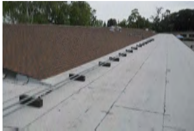
Roof Overview - Building 2 (Building 1, 3, 4, 5, 6 Similar)
