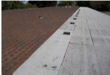
Roof Overview - Building 1
