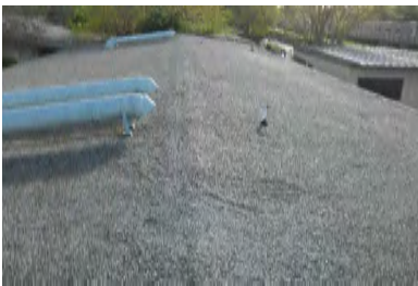
Roof Overview - Building 7
