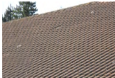
Roof Overview - Building 1100
