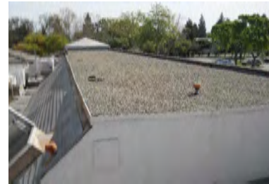
Roof Overview - Building 1100
