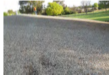
Roof Overview - Building 1
