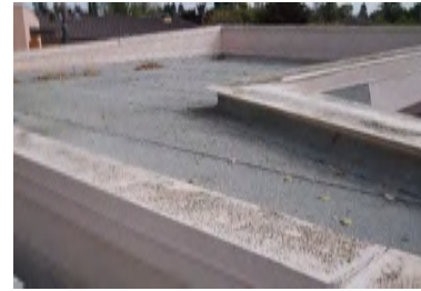
Roof Overview - Building H
