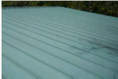
Roof Overview - Building A
