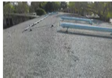
Roof Overview - Building 8
