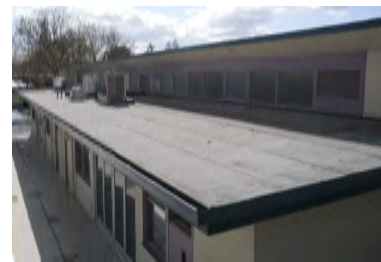
Roof Overview - Building 5 (Buildings 6 Similar)
