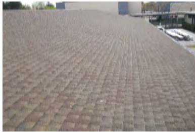
Roof Overview - Building H
