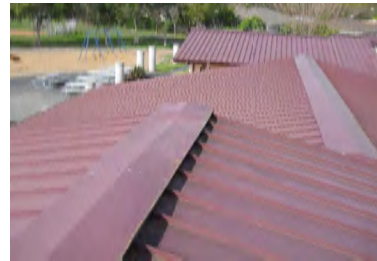
Roof Overview - Building E
