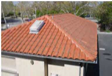
Roof Overview - Building 10
