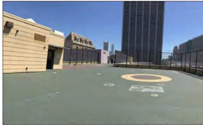
Rooftop Play Area at Level 4 with Storage and Stairs
