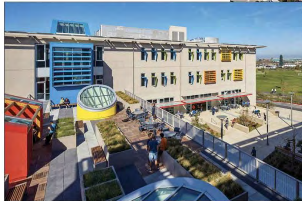
Rooftop Landscaped Terrace on Level 2
