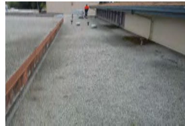
Roof Overview - Building 12
