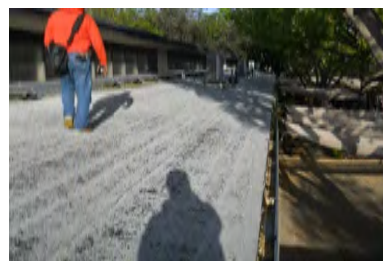
Roof Overview - Building 5 and 6 Similar
